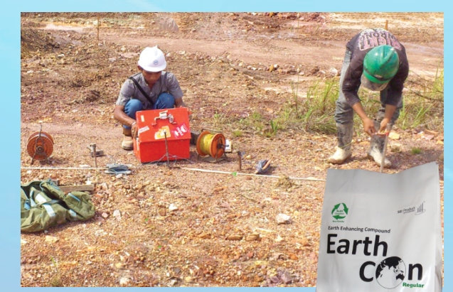
Professional Earthing System from SGI Engineers Pvt. Ltd.
